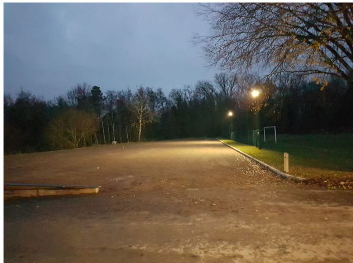
Eclairage parking SMA
